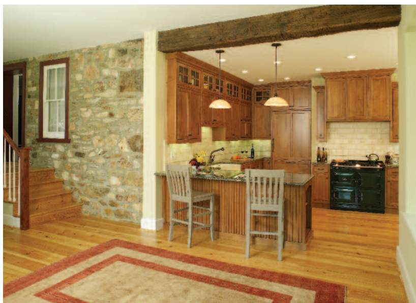
The re-pointed wall connects the new addition to the kitchen. Random-width pine flooring was used to unify the two spaces.
