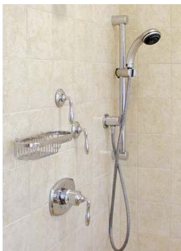
The plumbing fixtures are the Seabury series from Grohe. The Ginger shower baskets are attractive and the wire allows for easy drainage.
