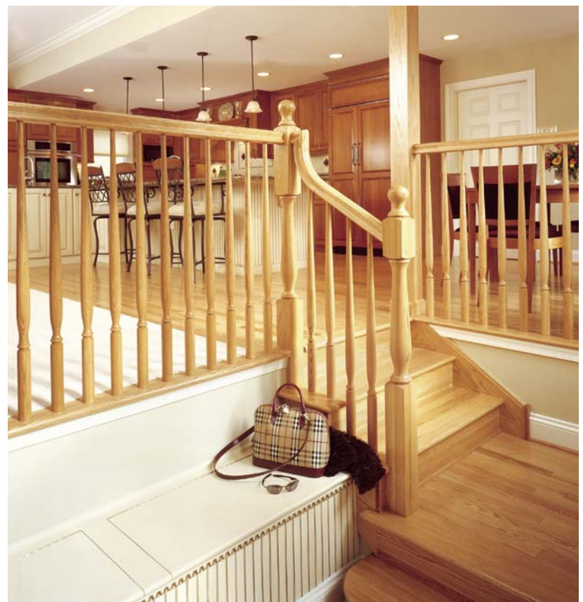
The oak post at the top of the stairs holds a beam that supports the second floor. It houses a convenient light switch and defines the entrance to the stairs. Photo by Ozzie, RVOiii Photography. rviiiiphotography.com
