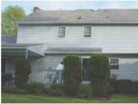
Left: A rear view of the home before the renovation.
