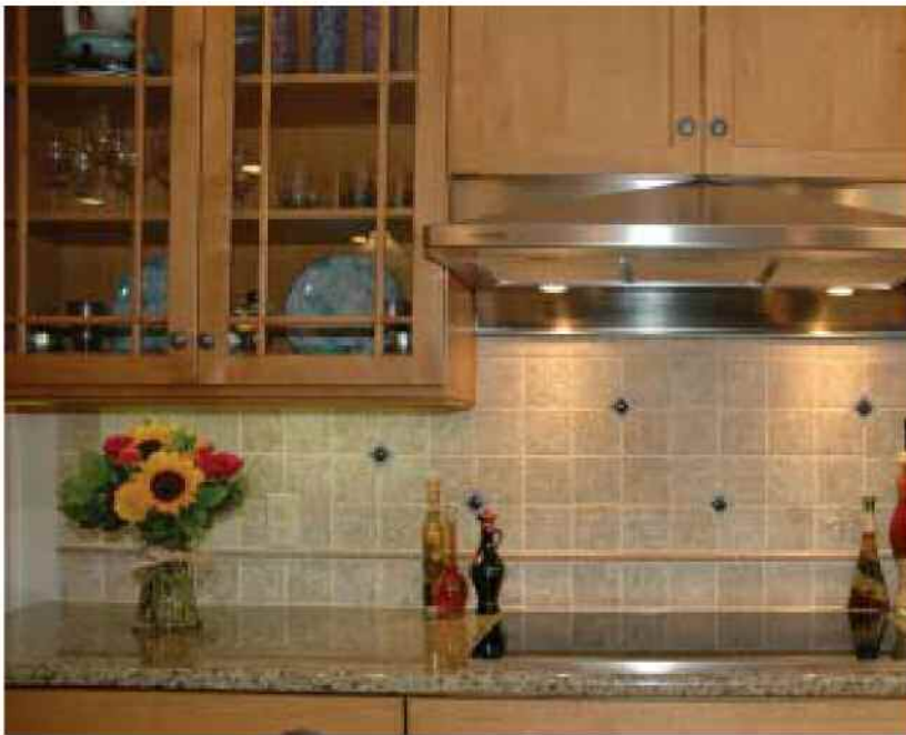
The backsplash, consisting of noche travertine tiles with 2-by-2 inch diamond-shaped aluminum pockets and handmade glass inserts, contains a splash of copper.
